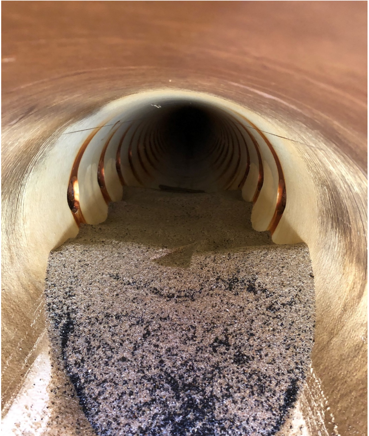
Underdrain – Train Six, Filter Eight.
