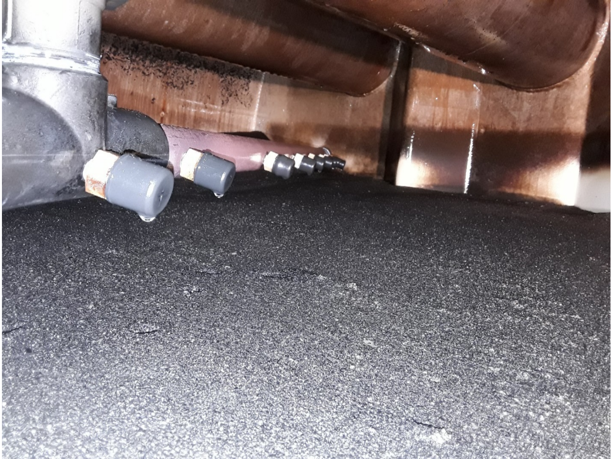
Cell B: Flat bed with 2" to 3" to the centerline of surface wash arms.
